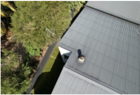
Roof Sheeting appears to be in reasonable condition
