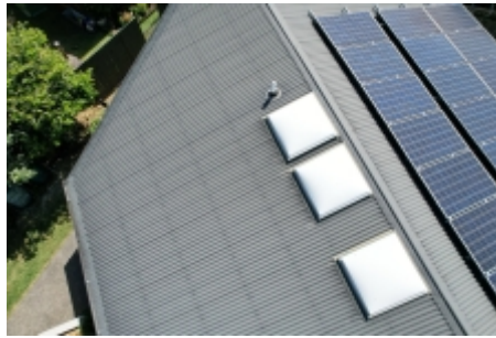
Roof Sheeting appears to be in reasonable condition
